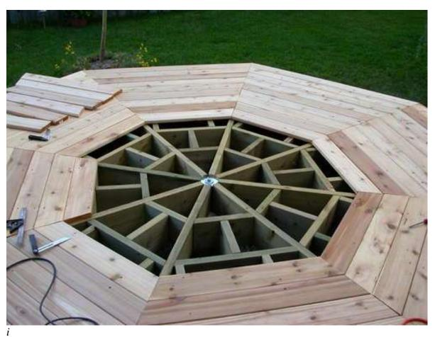
Start at the outer edge of the deck and work inwardly to the centre. The first row of decking overhangs the end joists by 1-1/2 inches.
