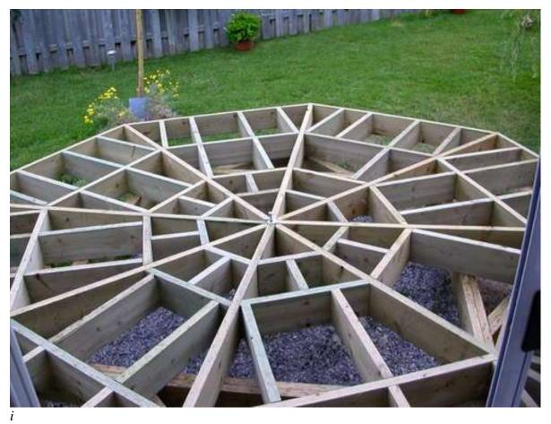
The Cross joists are perpendicular to the end joists are are set at 16 inch centres. Notice that the joists are clamped at the centre. This matrix of Joists, End Joists and Cross joints is extremely strong. Can you see the last one I was about to install, which ends the task of installing the joists for the deck? all joists are secured with deck screws.
