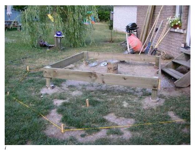
With the concrete firm, use 3 inch deck or brass screws to fasten a pressure treated 4"x4" upright in each of the 8 saddles. These uprights are marked and cut so that the top of each is level with the centre post. Screw pressure treated planks to the uprights to form a rectangle flush with the top of each upright.
