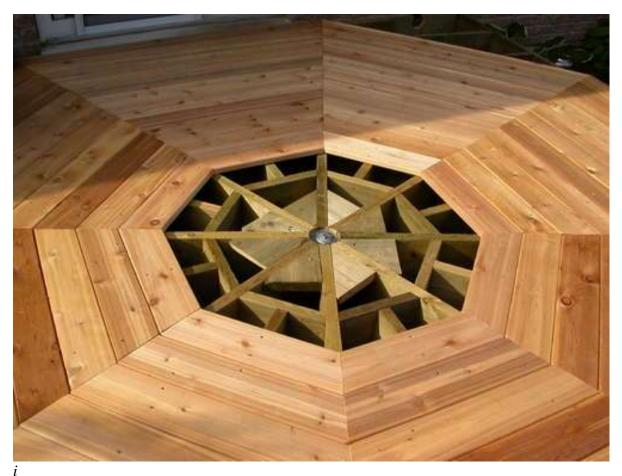
As you get closer to the centre of the deck, you will need to insert some scrap joisting to provide a surface to mount the decking. Additionally, since the deck planking is firmly holding the joisting together, we have the opportunity to modify the centre post clamping screw to asure that the final pieces of decking can be fastened in the centre, without interference.
