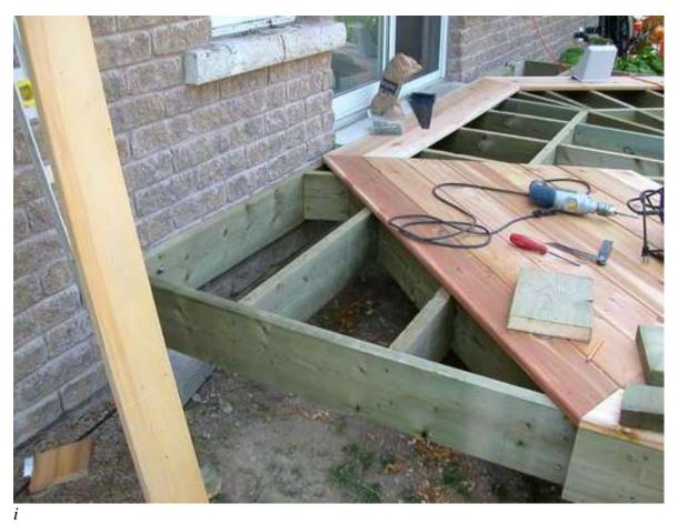
The connection of the Octagon deck to the house, required a small alteration in the plan. Keep the octagon shape, but deck the space between the wall and the deck and make it obvious. Here is the framing between the deck and house.
