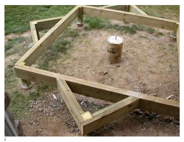
As in Step 5 the ODD numbered posts are framed to create a rectangle that intersects the rectangle of the EVEN posts. Follow the image, screw the pressure treated lumber in place and then double up the rectangles. What we have now is an 8 pointed polygon which is the deck foundation. Each Point or Vertex of the polygon will support a deck joist. (If you start the rectangle with the ODD numbered posts, it doesn't matter, as long as you end up with the 8 pointed polygon.)
