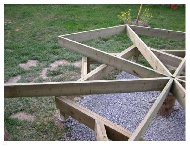
There are 8 main deck joists, each crossing a vertices and resting on the centre post, giving us a 2 foot cantilever to the deck. Each joist is 6 feet long and sits at angle of 45 degrees from adjacent vertices.
