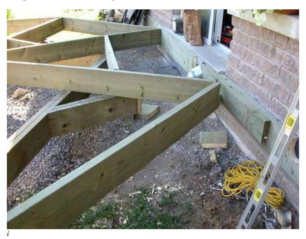
I used 2 ledger boards here to accomodate two vent pipes and to assure that I had a attachment surface beyond the entrance lintel.
